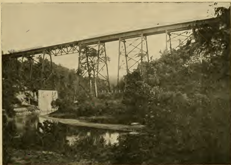
MARTIC FORGE RAILROAD BRIDGE
