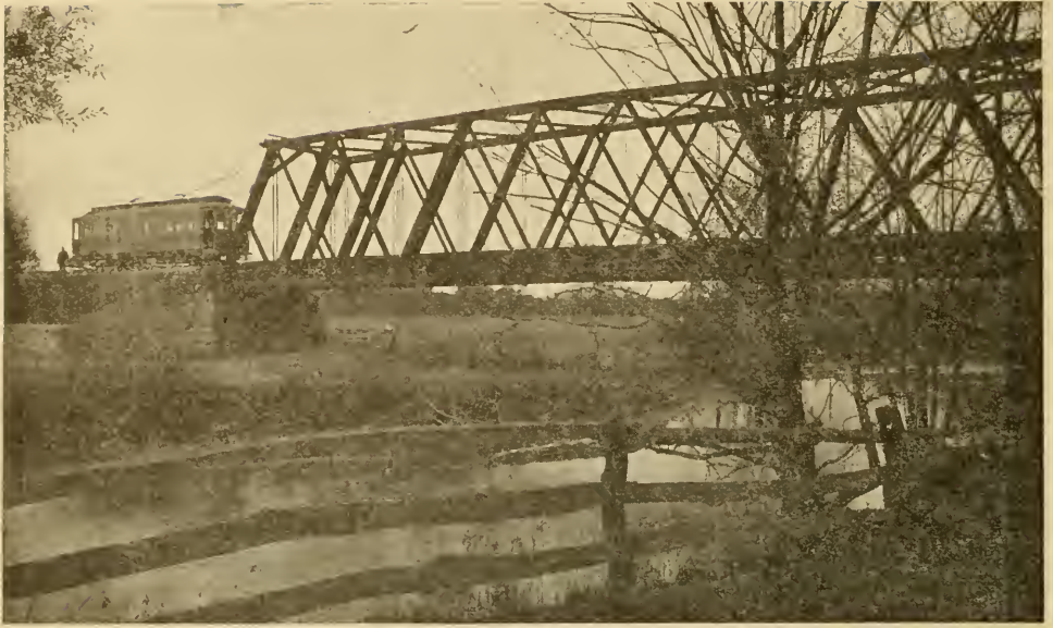
BRIDGE ACROSS THE CONESTOGA NEAR BLUE BALL
